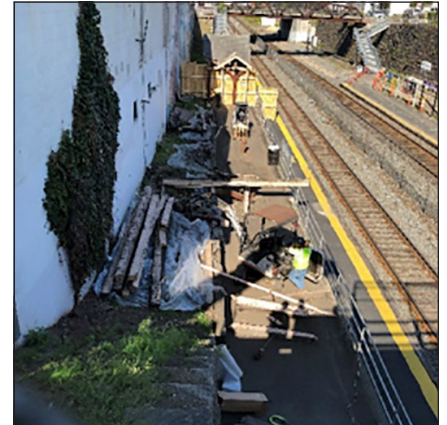
Completed demolition of the wood canopy on the inbound track platform.
