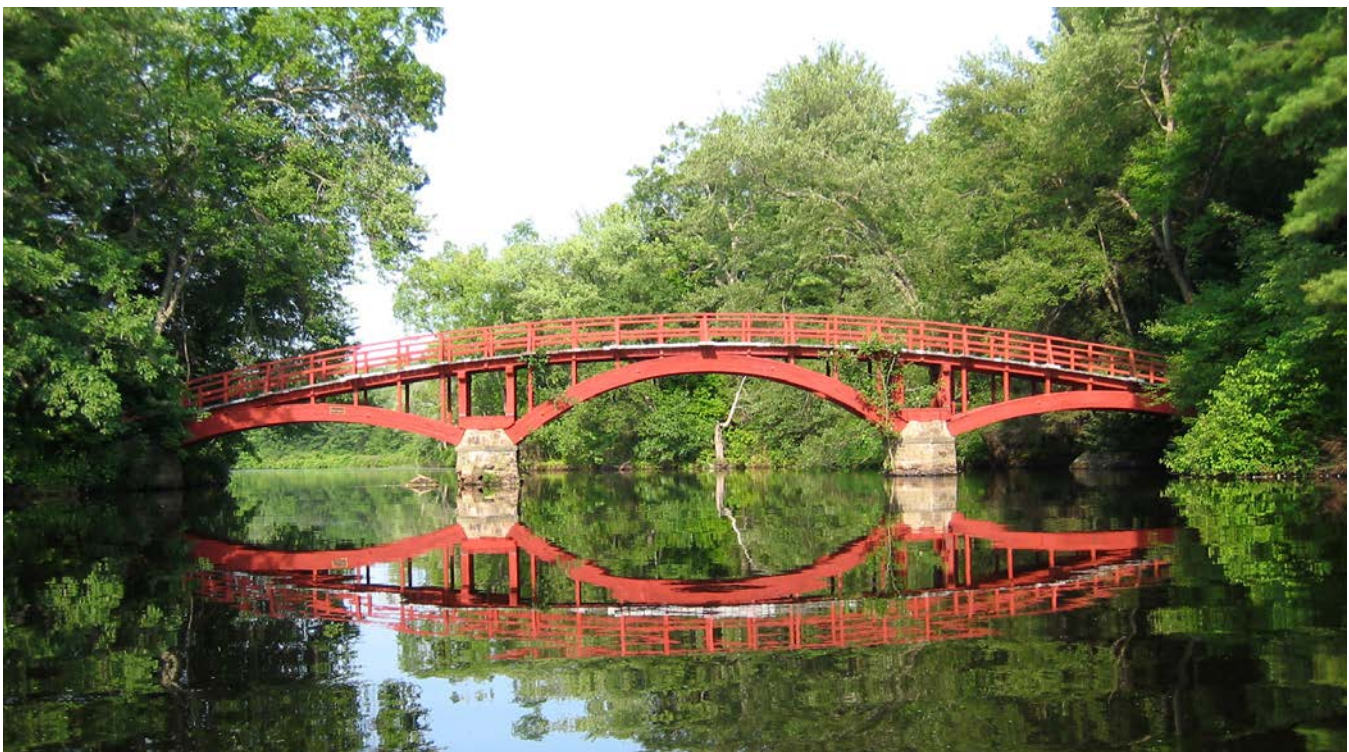
Red Bridge on Charles River | Photo: Martin Kessel
