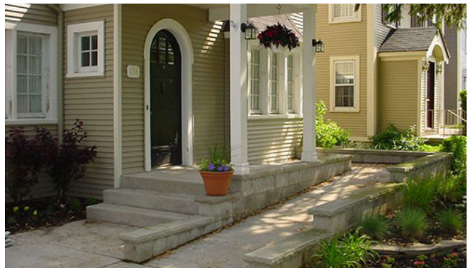
Accessibility retrofits to older single family homes Photo: IDEA Center, of Buffalo
