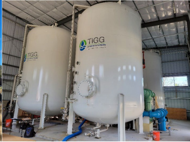
Newly Installed H&T GAC Filter Vessels
