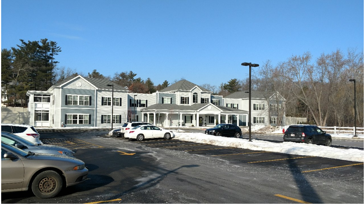
Reading Artis Building of 64 units (front view)
