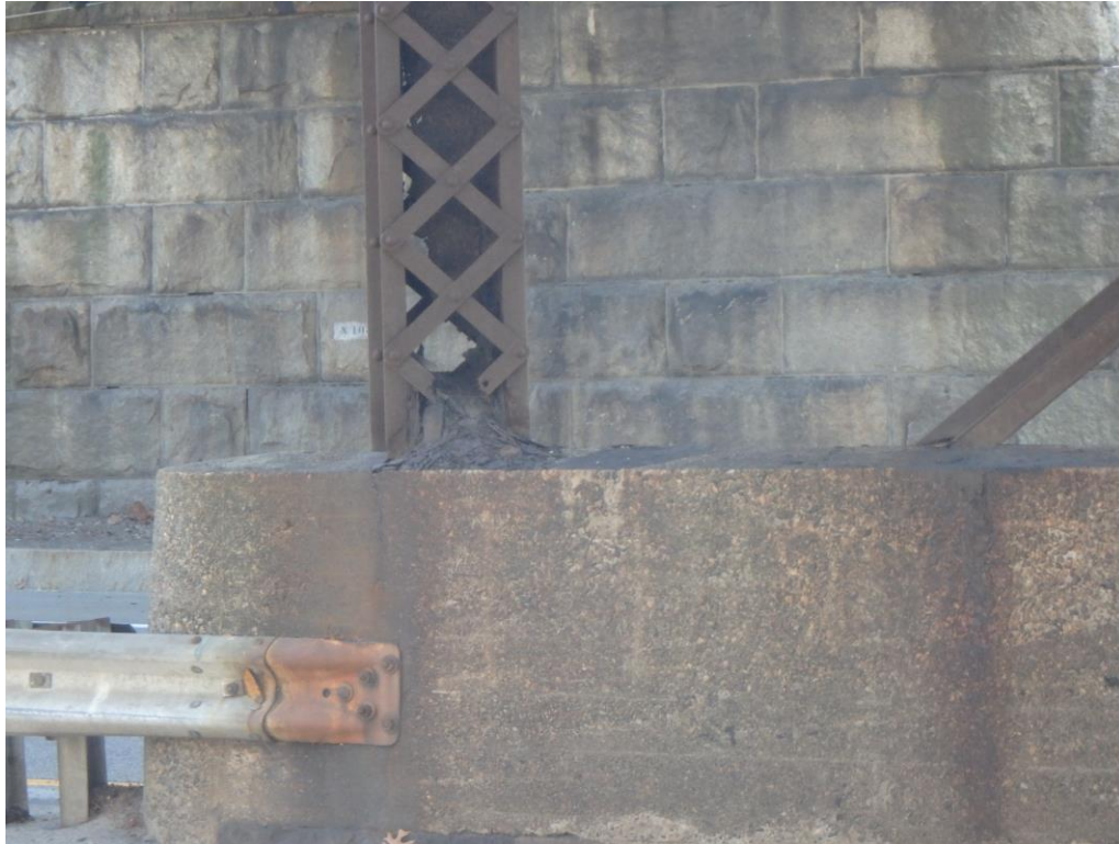
Typical Section Loss to Pier Column
