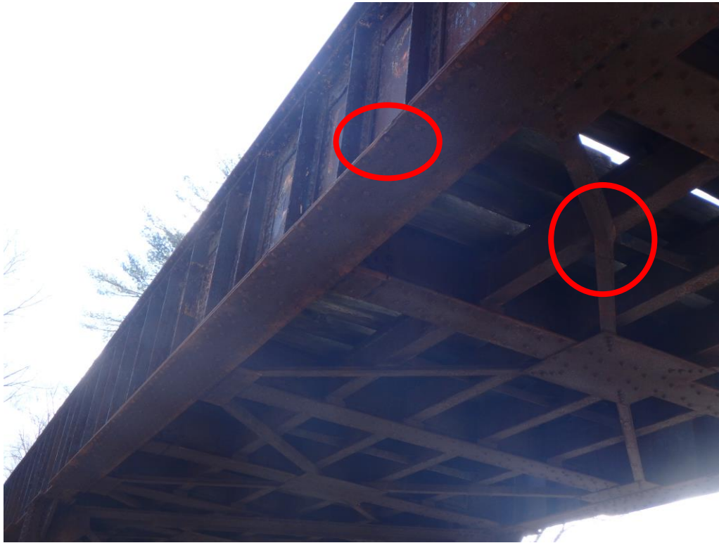
Collision Damage to East Girder and Diagonal Bracing
