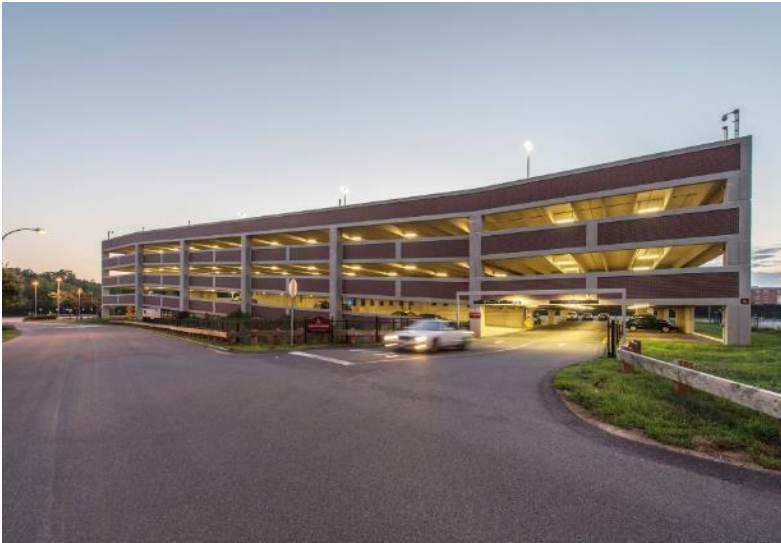
Thin-Brick Integral with Precast Exterior Beams
