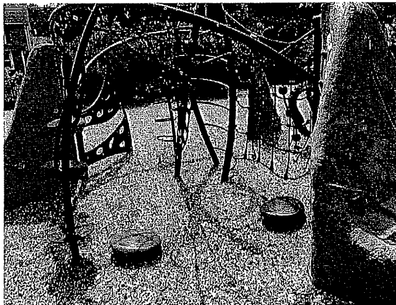
Johnson School Space Walk – 2 broken pods on ground Manufacturer - Play and Park
