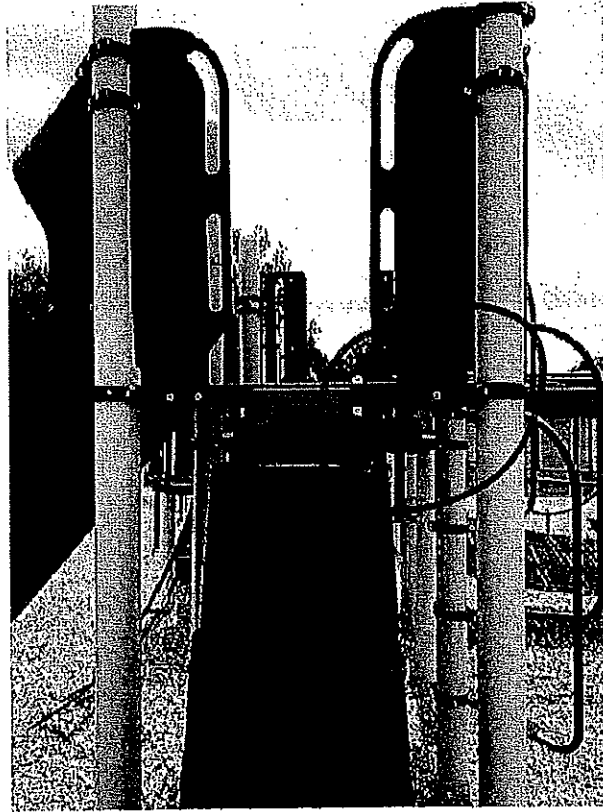
Memorial School (Front) Replace Missing Bolt (circled) Manufacturer – Landscape Structures
